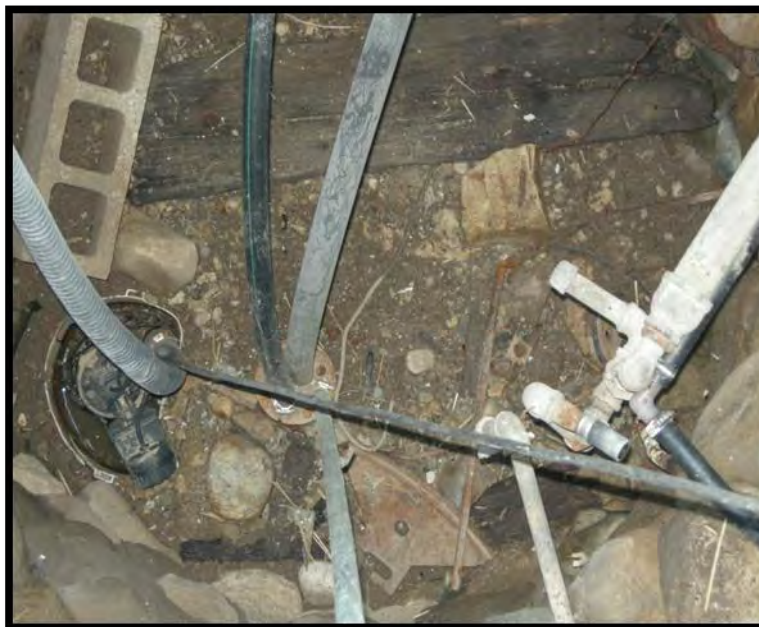
Figure 4: Poorly maintained wells can provide a conduit for contaminants to travel from the surface down to the aquifer. (SGSNBP Source Protection Region)
