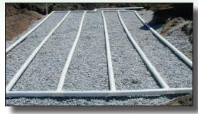
Septic systems — including leaching beds — need to be designed properly to protect water and need to be maintained properly and inspected.
